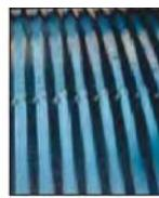
**6.** The liner is suspended inside the tank to form a water-tight membrane. Water never contacts the tank's steel surface.
