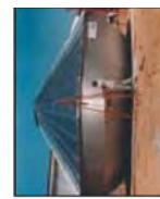
**8.** All steel components are hot-dipped in zinc for high corrosion resistance. SCAFCO's unique 42 2/3" galvanized steel side-wall staves are pre-punched with a single stroke operation, assuring accurate hole alignment. Sheets are precision roll-formed from high-strength steel. Our extra-stiff 2 1/3" corrugation provides resistance to wind loads. The tank can be field painted if the owner desires.
