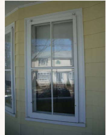
A traditional wood storm window fastened by hangers at the top. This storm window is also secured by four screws along the perimeter.
