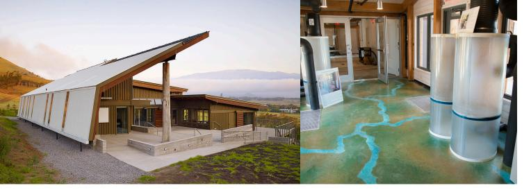
The roof and north facade of the Energy Lab at Hawai'i Preparatory Academy are designed to capture fog through condensation that flows to a gutter at the base of the facade wall and then to the 10,000-gallon cistern.
